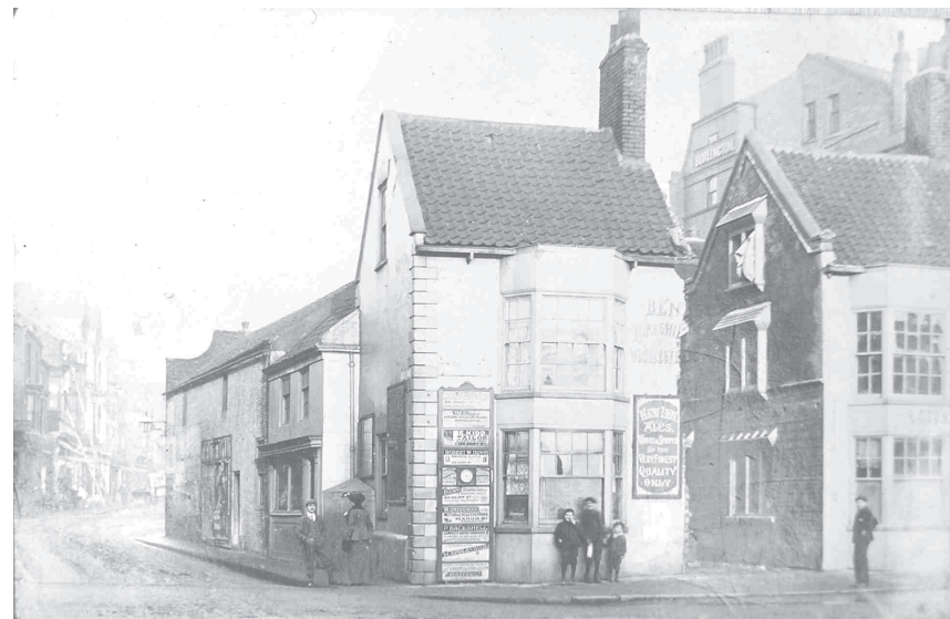
Preparing to widen Cross Street. The New Inn is sliced through and a new gable end erected. Soon after this photograph was taken the left hand side was demolished.
